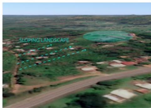
The site is located on a slight grade leading up to a hilltop. With this in mind, the team coordinated building types to meet the slope requirements and allow maximum circulation. Additionally ADA ramps were placed strategically to accommodate every need equally.
